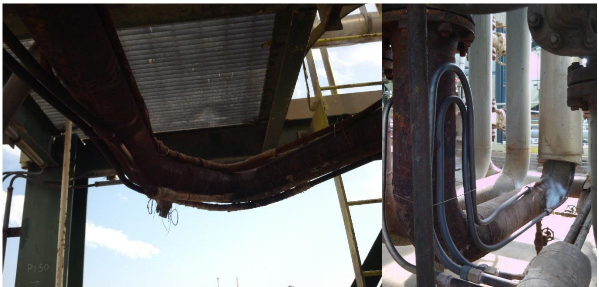
Figure 6. Sour water acid gas piping tracing.
