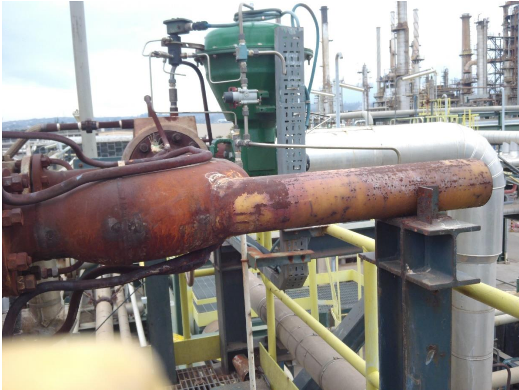
Figure 7. Tracing of vent gas piping including unheated pipe support.
