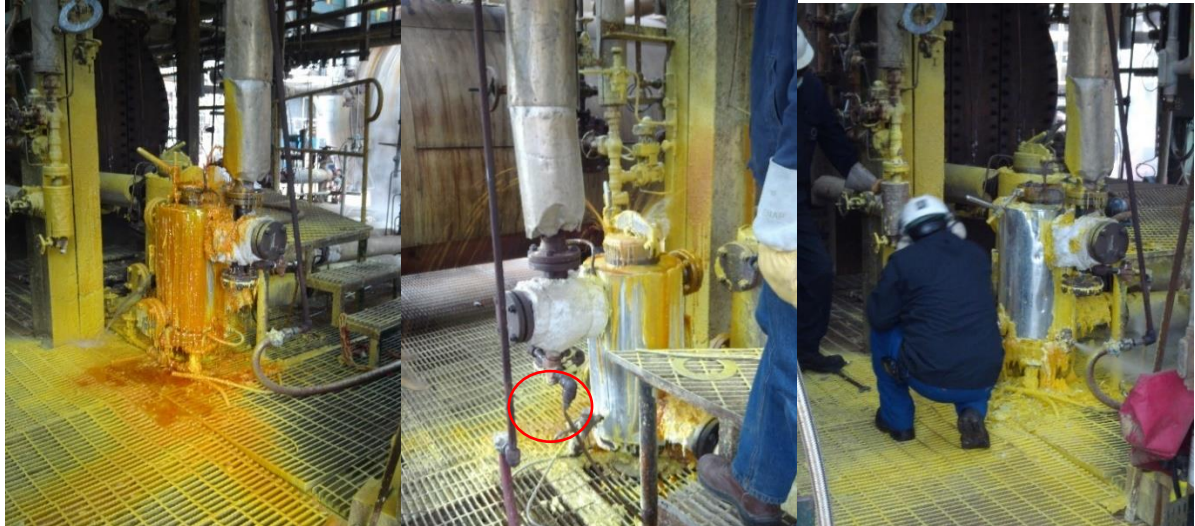
Figure 9. Consequences of frozen Sultrap in URA1.
