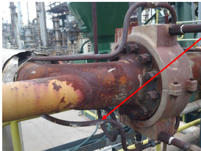
Figure 8. Bolt-on jacketing for flanges.
