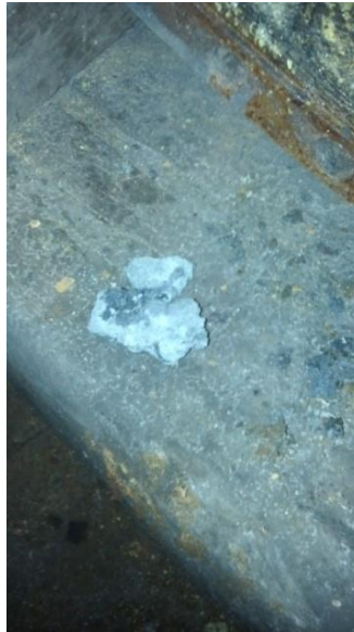
Figure 23 - Foreign Material in the Outlet Channel of the Second Condenser
