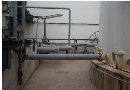
Figure 17. Amine Surge/Storage Tank inlet and outlet nozzle
