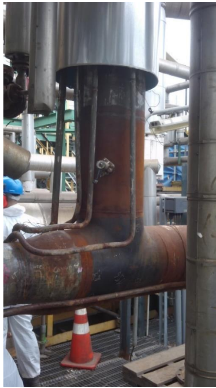
Figure 5. URA2 Tail gas piping tracing.
