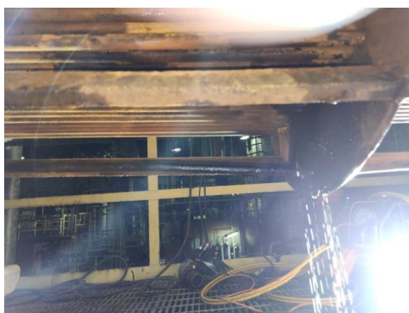
Figure 34 – Tube Failure: Second Reheater after removal of the tube bundle
