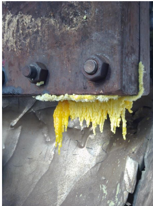
Figure 15. Evidence of sulfur from the demister box in URA2 Third Condenser C-1644
