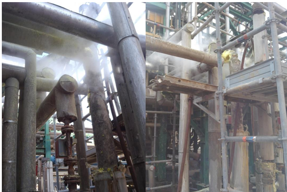
Figure 3. Vent air escaping from the access hatches in URA3 Sulfur Pit
