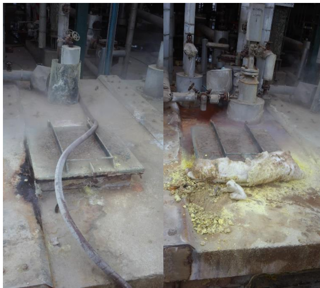
Figure 3. Vent air escaping from the access hatches in URA3 Sulfur Pit
